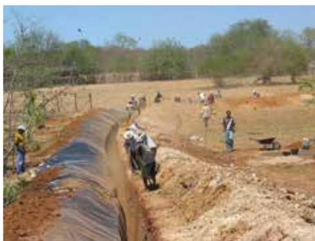
**Figure 5** Building a sub-surface dam
