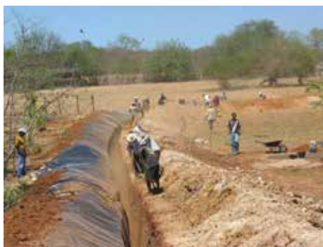
Figure 5 Building a sub-surface dam
