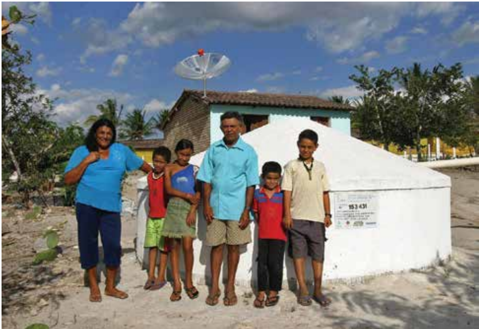
Figure 3 A drinking water cistern constructed by ASA
